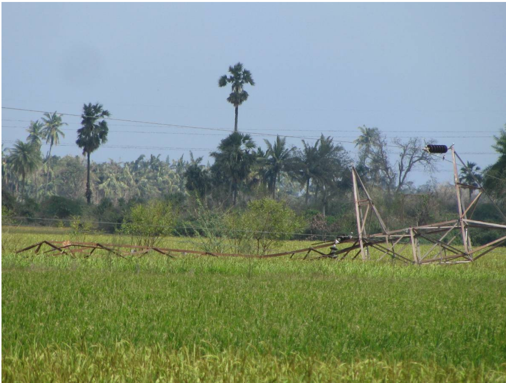
Damage and rectification work in Sornavur - Nallathur 110 KV line
