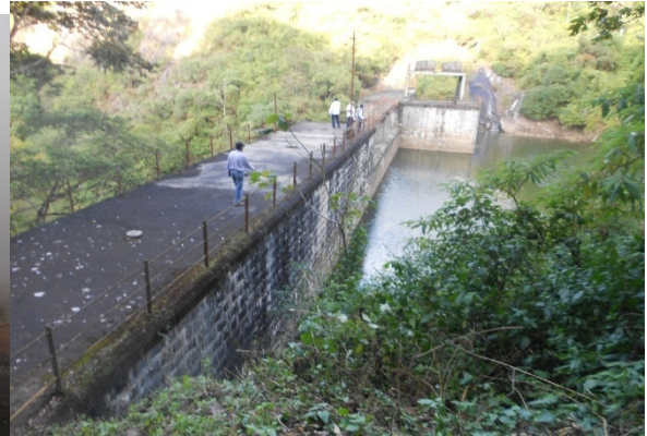
Upstream face of dam with leaching
