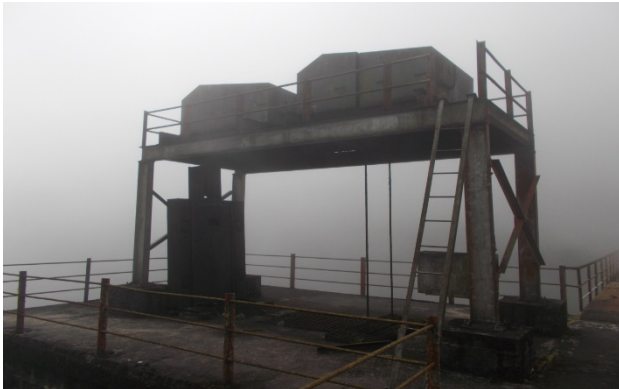
Rusted/worn out hoisting mechanism, steel wire ropes, gates and hoist supporting structure of scour vent gates.
