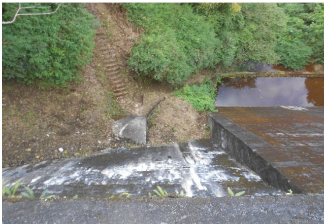
Downstream face of dam with leaching
