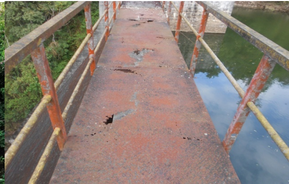
Damaged spillway steel Deck Bridge
