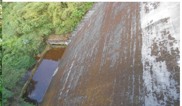
Formation of algae on the downstream face of spillway glacis and abutment
