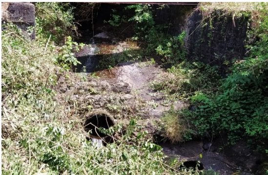
Damaged masonry wall with RCC plume pipe location
