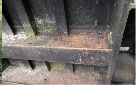
The rusted scour vent gates
