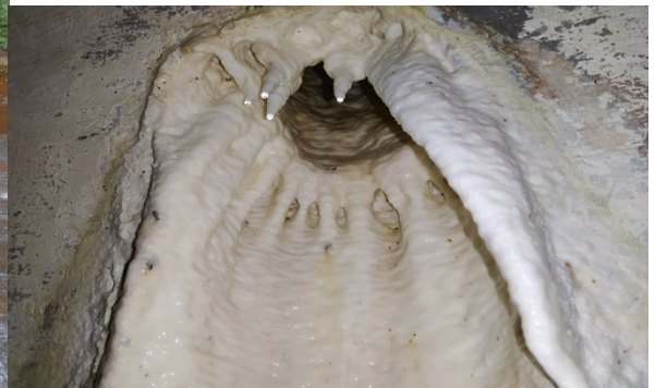
Calcinations deposition at vertical shaft holes
