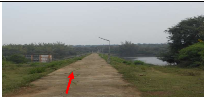
Longitudinal crack on the concrete layer of Earthen Dam
