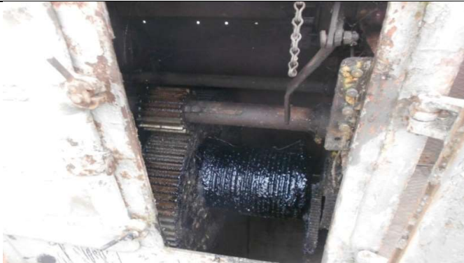
Scour vent gate hoisting arrangements.
