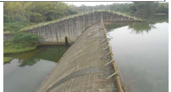
Damaged flash board on top of Spillway and calcination of the right flank guide wall
