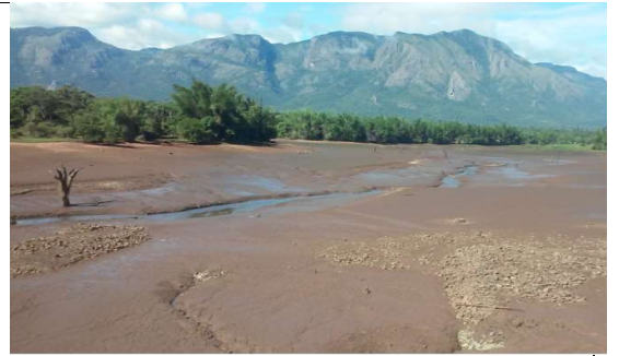
Sedimentation inside the reservoir observed during August / 2020 depletion
