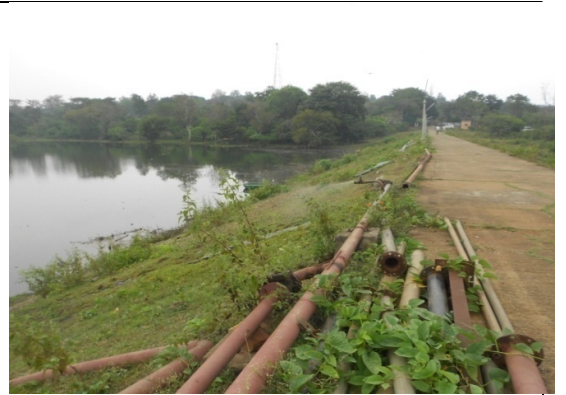
Damaged water supply line from the reservoir to Camp.
