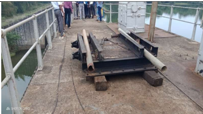
Damaged intake gate.
