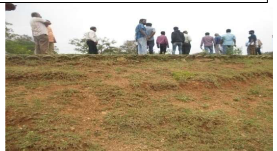
Damaged earthen bund on the upstream side
