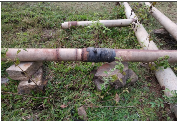
Damaged water supply line.
