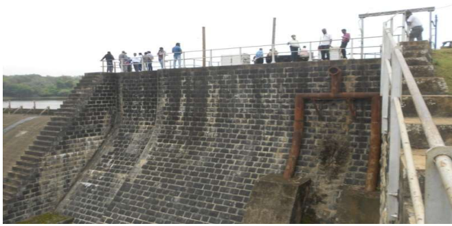
Calcination deposit on the downstream side of Dam masonry
