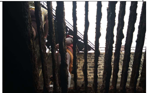
Damaged trash rack panels of intake gate.
