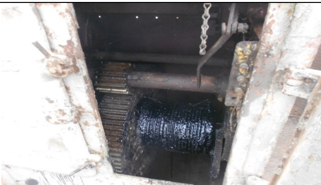
Scour vent gate hoisting arrangements.
