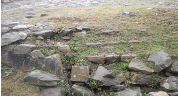
Disturbed rock toe of earthen bund on the downstream side
