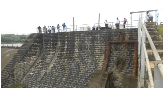
Calcination deposit on the downstream side of Dam masonry
