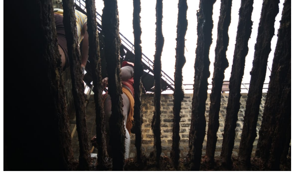
Damaged trash rack panels of intake gate.
