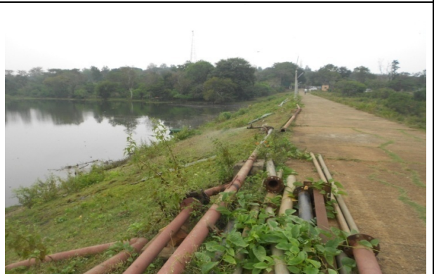
Damaged water supply line from the reservoir to Camp.
