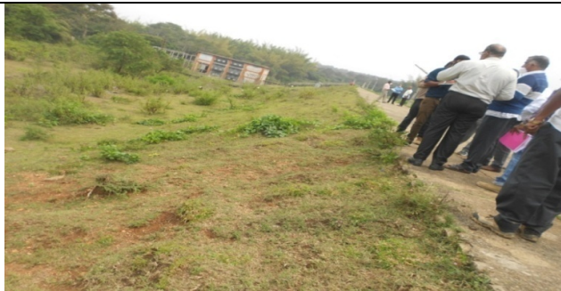
Damaged earthen bund on the downstream side - Proper slope to be restored
