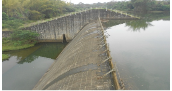
Damaged flash board on top of Spillway and calcination of the right flank guide wall
