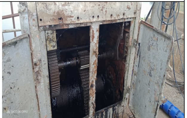
Intake gate hoisting arrangements
