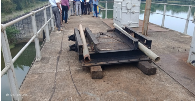
Damaged intake gate.
