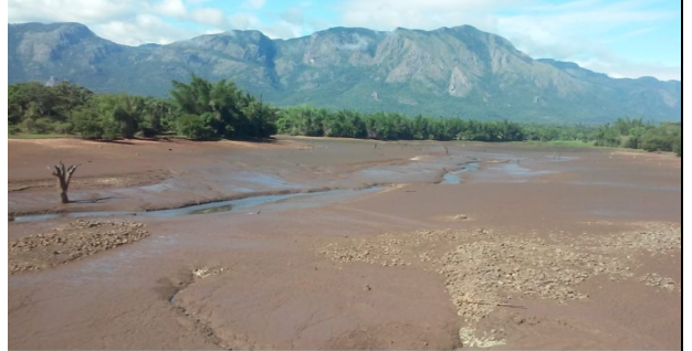
Sedimentation inside the reservoir observed during August / 2020 depletion
