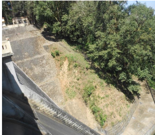
The left flank D/S earth portion without having protection from the slip
