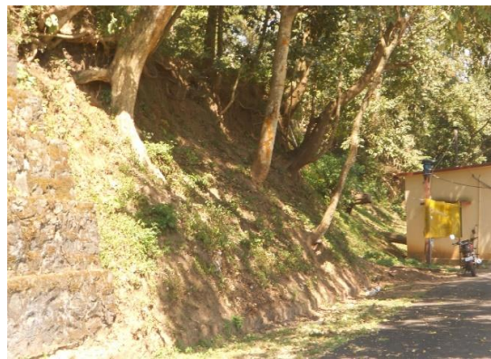
The earth slip adjacent to the slope protection work.
