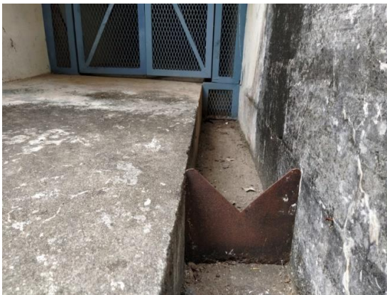
Gallery gate and the V notch fixed in the seepage outlet drain
