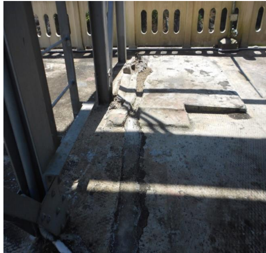
Screed concrete has been proposed to rectify the defects.
