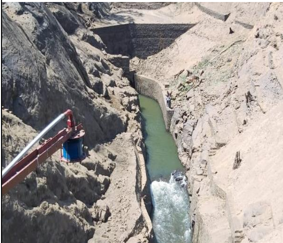
Damaged condition of the slope protections on the left flank of the offtake channel from the tunnel
