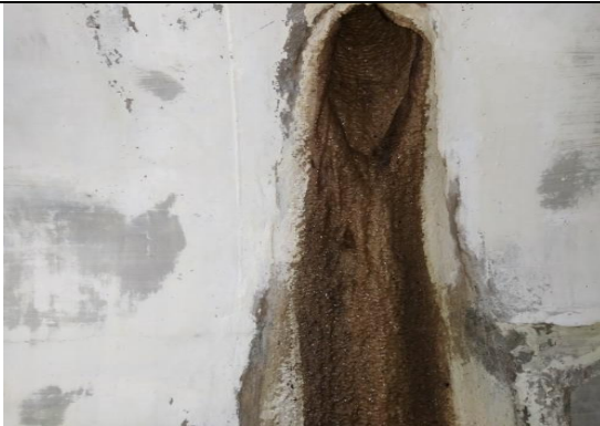
calcinations deposits at vertical shaft holes
