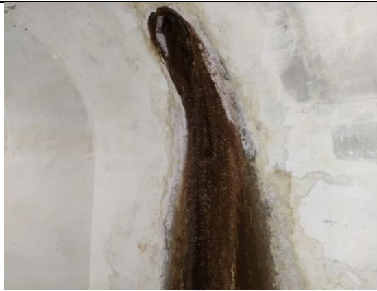
calcinations deposits at vertical shaft holes
