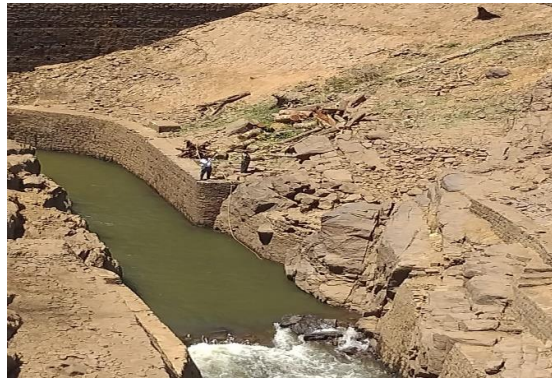
Damaged condition of the slope protections on the left flank of the offtake channel from the tunnel
