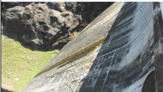
Water oozing on left flank downstream side
