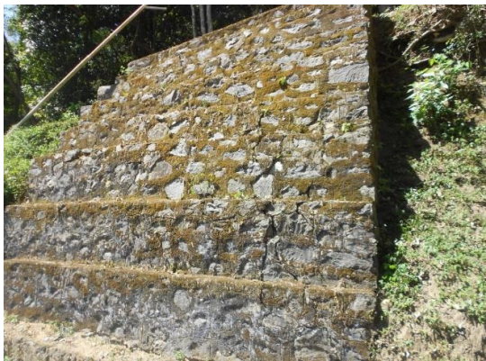
damaged condition of slope protection works of the approach road due to the non-provision of weep holes
