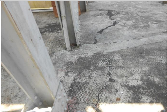
Screed concrete has been proposed to rectify the defects.
