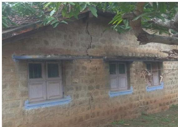
The dilapidated condition of 2 AE type quarters and Civil office at Periyar lower camp
