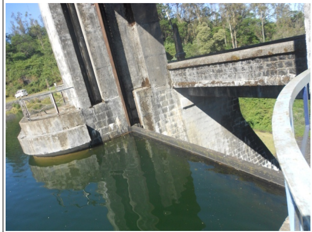
SPILLWAY GATE SKIN PLATE TO BE REPLACED
