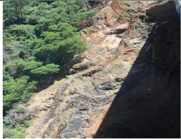
DOWNSTREAM RIGHT FLANK STEPS TO BE RECTIFIED
