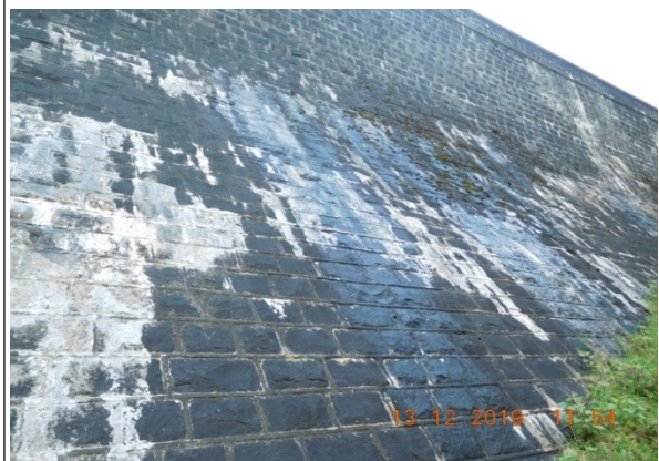
DOWNSTREAM LEFT FLANK LEACHING
