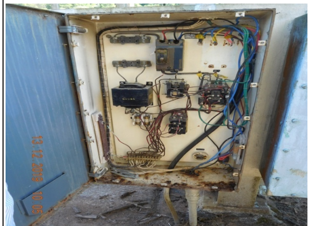
SCOUR VENT GATE CONTROL PANELS AND CABLES TO BE REPLACED
