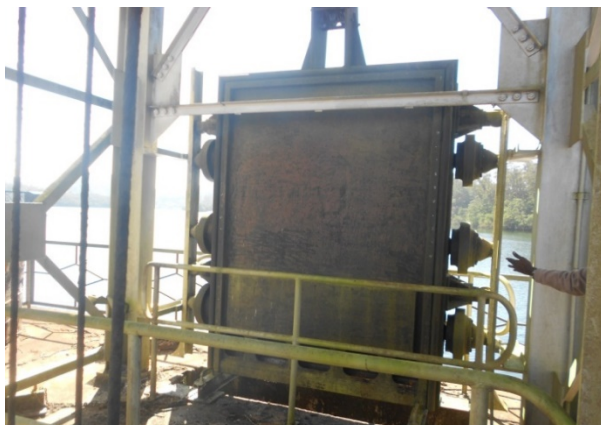
SCOUR VENT GATE AND ITS HOISTING MECHANISM TO BE
