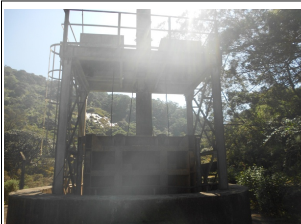
POWER INTAKE EMERGENCY GATE AND ITS HOISTING MECHANISM TO BE OVERHAULED
