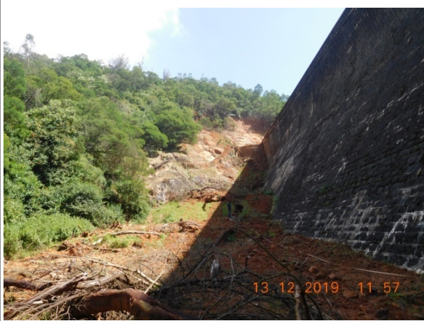
DOWNSTREAM RIGHT FLANK SIDE SLOPE AREA DEBRIS TO BE CLEARED AND PROTECTED
