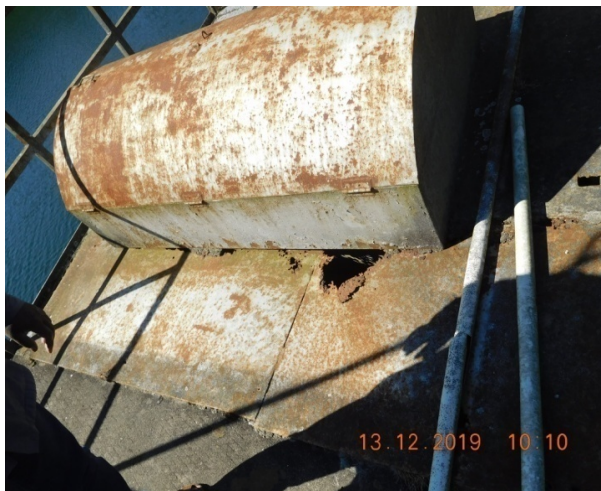
HOISTING PLATFORM CHEQUERED PLATE TO BE REPLACED
