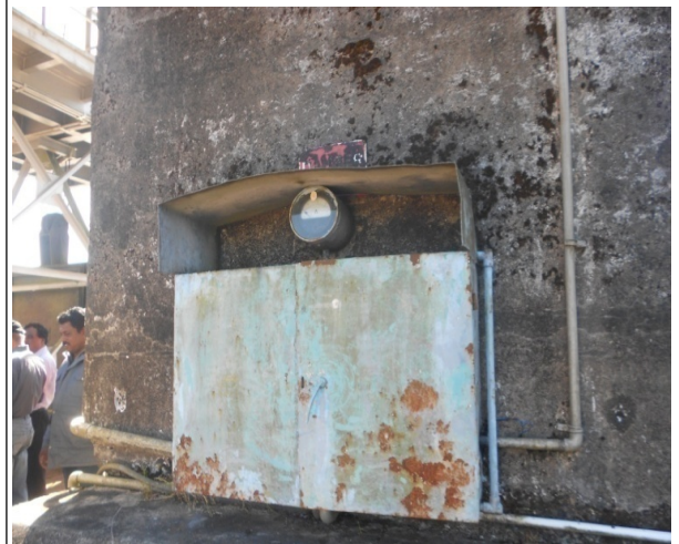
SPILLWAY GATE CONTROL PANELS AND CABLES TO BE REPLACED
