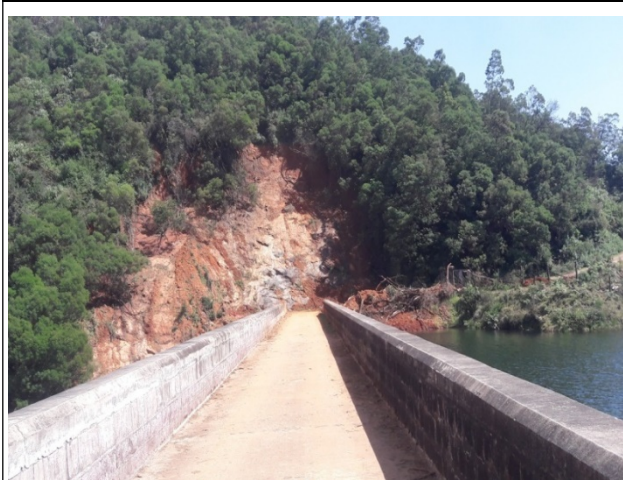
EARTHSLIP NEAR DAM RIGHT FLANK
