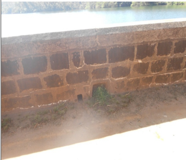
DAM TOP TO BE SCREED CONCRETED FOR PROPER DRAINAGE
