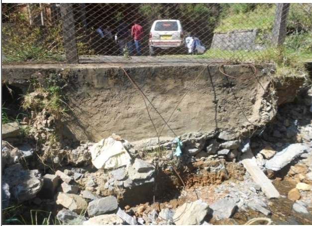
CONCRETE AROUND POWER INTAKE SERVICE GATE WELL TO BE RECTIFIED
