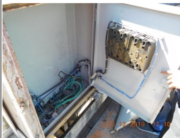
POWER INTAKE CONTROL PANELS AND CABLES TO BE REPLACED
