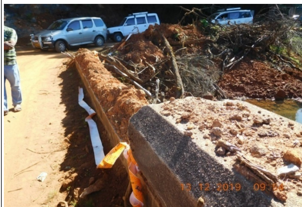
DAMAGED RIGHT FLANK DAM TOP PARAPET WALLS
