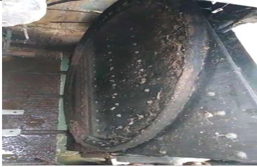
Damaged seal of intake gate
