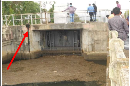
Steel wire rope and screw rod mechanism of scour vent gate
