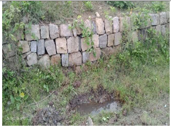
Seepage observed location on the right flank side near check post
