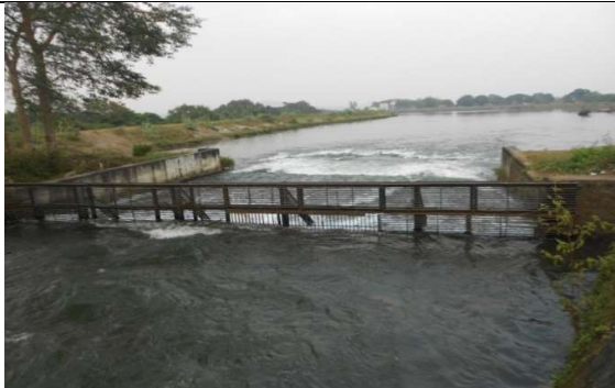
Rectification work on the both side of trash rack
