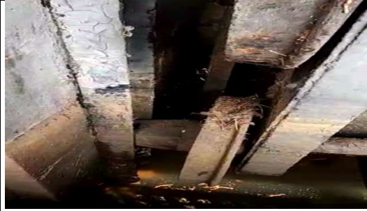
Intake gate guide rollers in jammed and rusted condition
