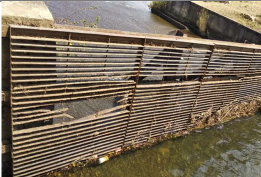
Damaged trash rack panels at flume exit (04.11.2020)
