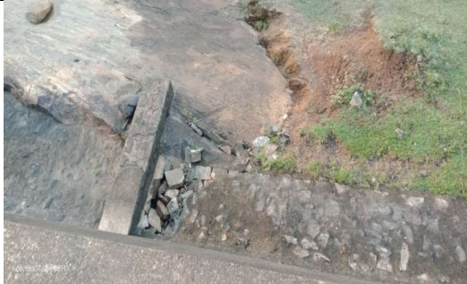
Damaged pitching portion on the downstream side of the Spillway
