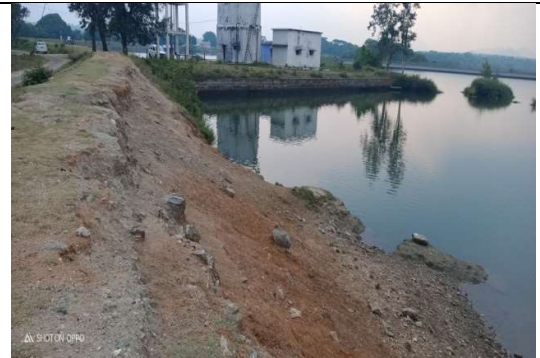
Damaged right flank bend near the Check post
