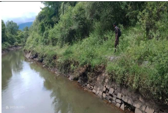
Damaged lining portion of flume (Maravakandy Dam to Moyar Forebay Dam)
