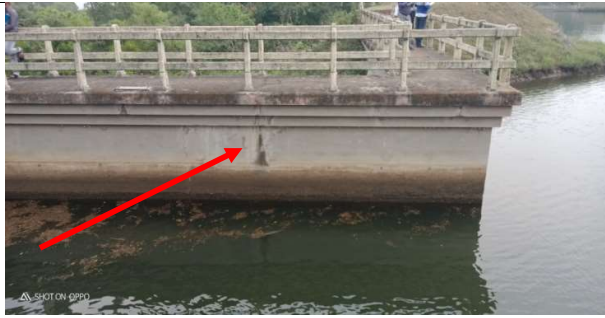
Hairline cracks on the upstream side of concrete dam near intake.
