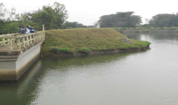
Unprotected upstream bund portion near intake
