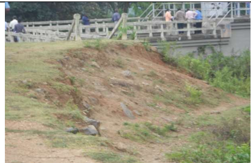
Damaged bund portion on the downstream side near intake
