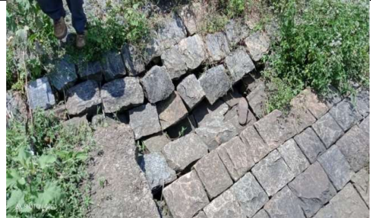
Dislocated pictching near flume exit point
