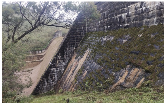
Downstream face with calcium leaching with algae growth
