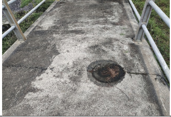
Vertical shafts without proper cover
