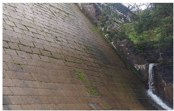
Spillway with algae growth
