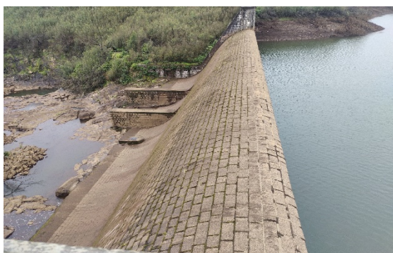
Spillway with algae growth
