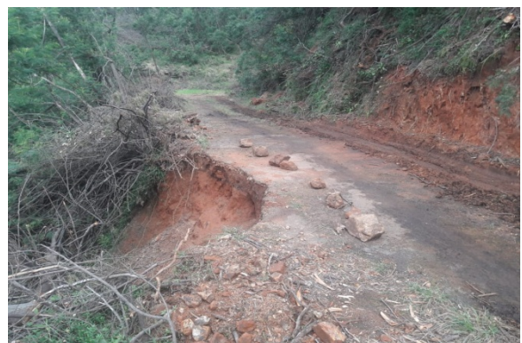
Damaged BT surface and slipped earth
