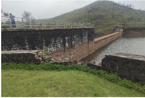
Damaged RR Protection Wall on the Left Flank side
