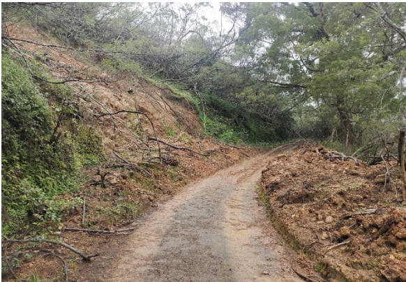
Damaged BT surface and slipped earth
