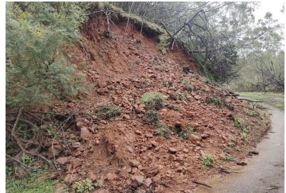
Damaged BT surface and slipped earth
