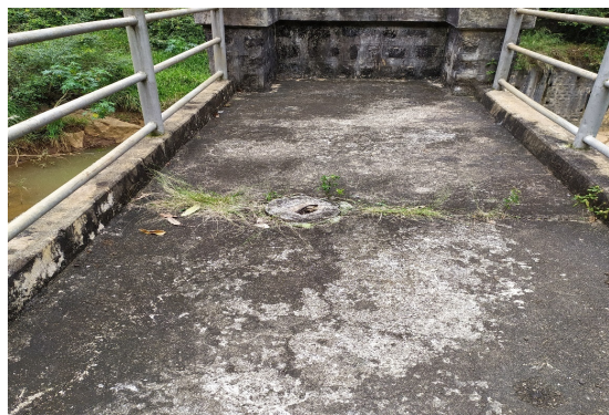
Chocked Vertical shaft of Weir
