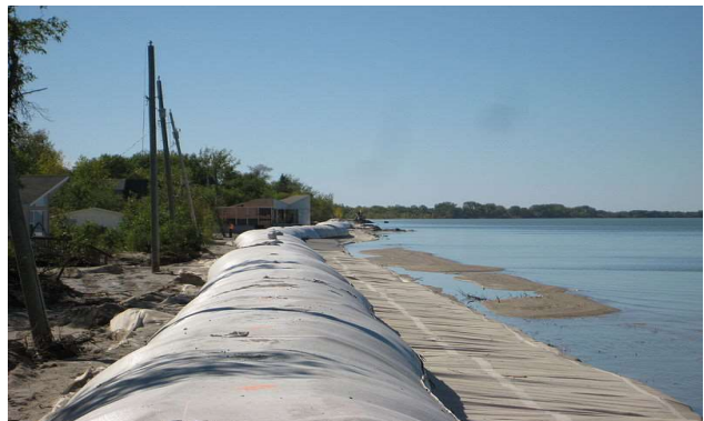
Geotextile tubes being filled with sediments.
