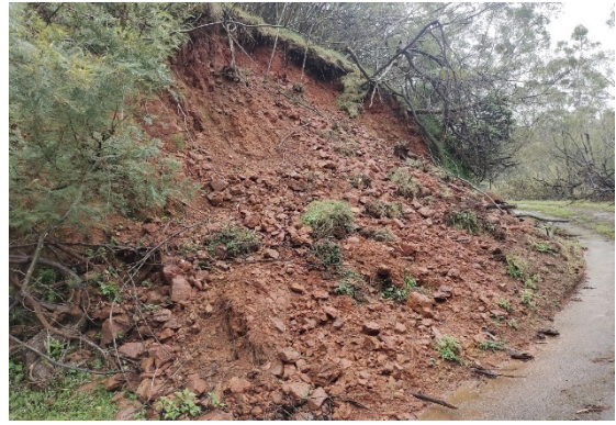
Damaged BT surface and slipped earth
