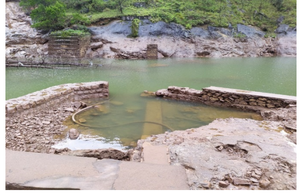
Cavity portion filled with lean mixed concrete
