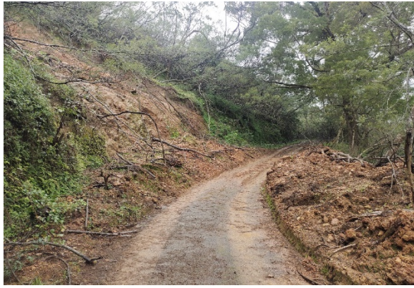
Damaged BT surface and slipped earth
