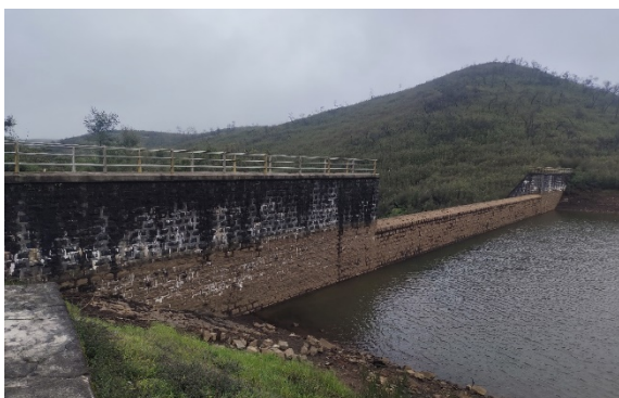
Damaged RR Protection Wall on the Left Flank side
