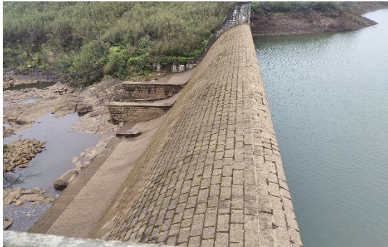
Spillway with algae growth
