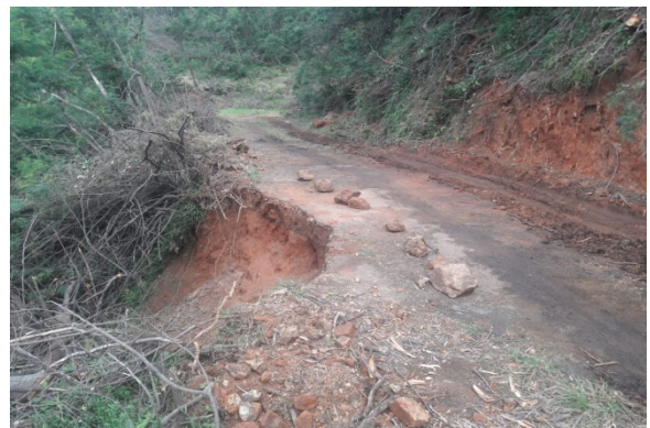
Scoured road side require to be protected
