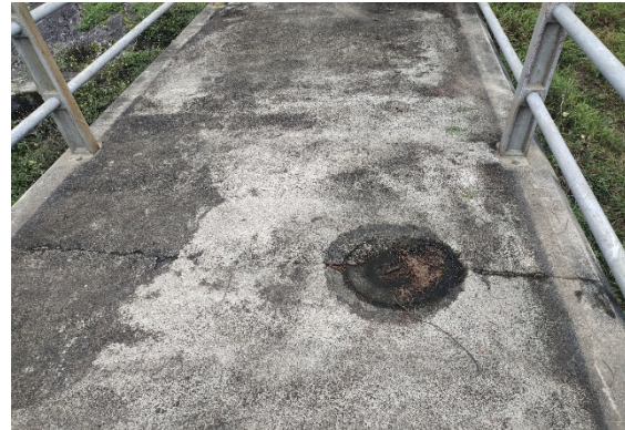
Vertical shafts without proper cover
