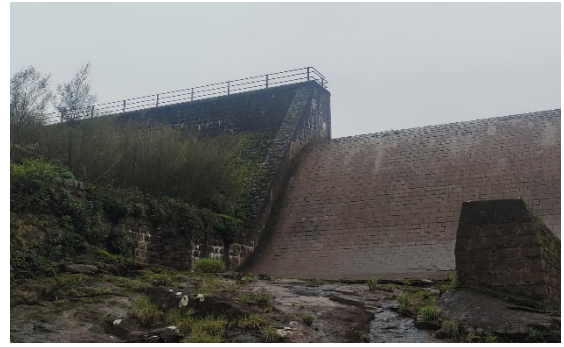
Downstream face with calcium leaching with algae growth
