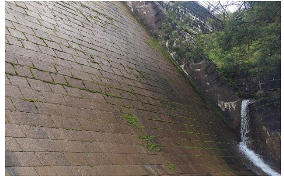
Spillway with algae growth
