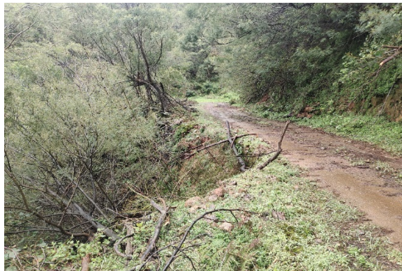
Scoured road side require to be protected
