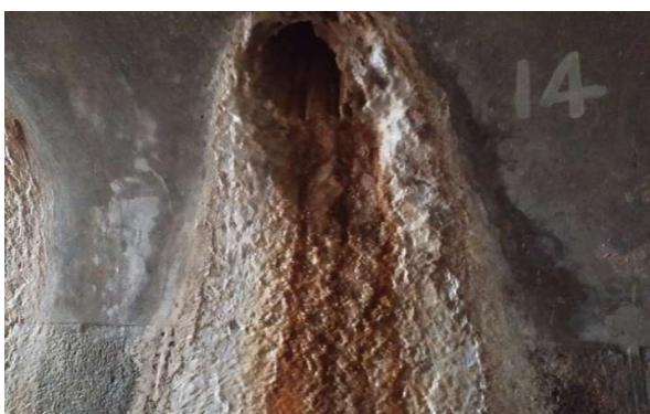
Calcination through Vertical shaft inside Drainage gallery
