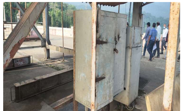
Outdated / Worn out control panels of Intake Gates
