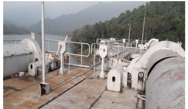
Rusted / corroded hoisting platform of intake gates
