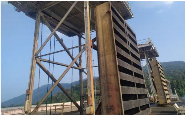
Rusted intake gate structure
