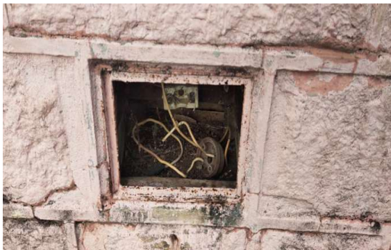
Worn out wiring system at Dam top
