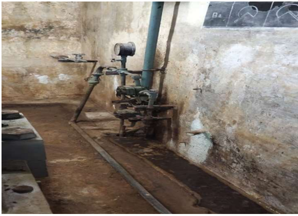
Outdated and deteriorated hydraulic seal arrangements of radial Scour Vent Gate
