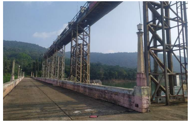
Rusted Spill Way Gate structure and its platform
