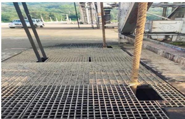
Worn out steel wire ropes of Intake Gate
