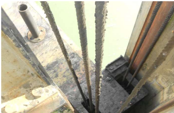
Worn out steel wire ropes of Spill Way gate
