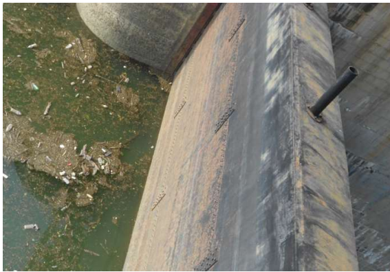
Rusted skin plate (upstream side) of Spill Way Gate
