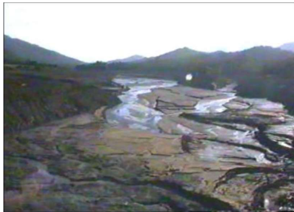
Slit deposition inside Pillur reservoir photographed during 1991
