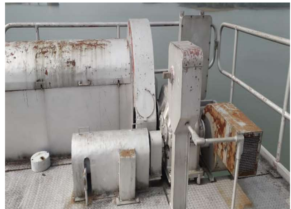
Rusted Operating Mechanism covers and air dampers of scour vent gate
