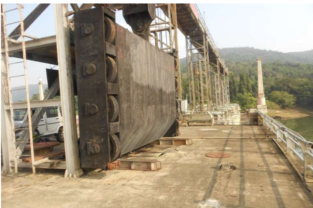
Rusted and Jammed Main Guide rollers of Scour Vent Emergency Gate
