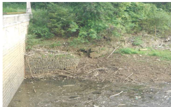
Right Flank slops near the dam to be rectified
