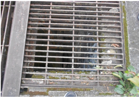
Intake gate needs to be Overhauled and Painted
