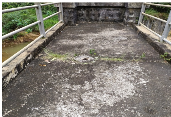
Chocked Vertical shaft of Weir
