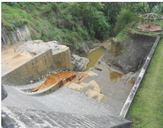
No approach to the Scour Vent Operating Platform
