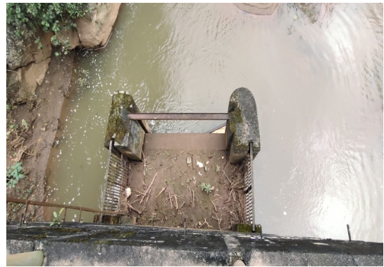
Worn out and Chocked Trash rack panels at Tunnel Intake
