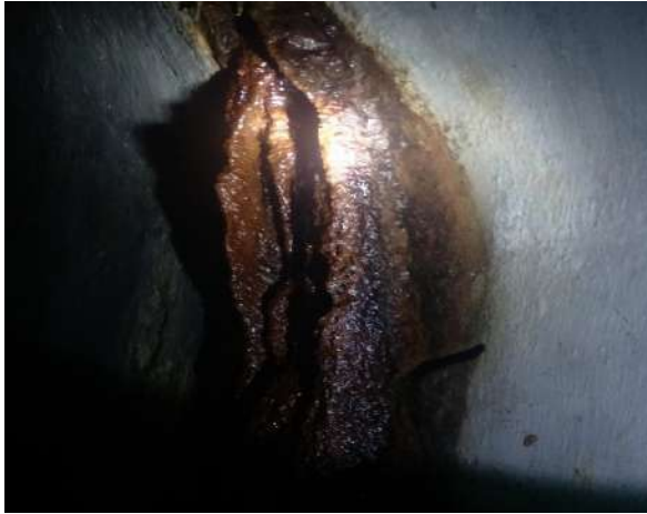
Earth Sludge coming out through Vertical shafts in Blocks 11 & 12
