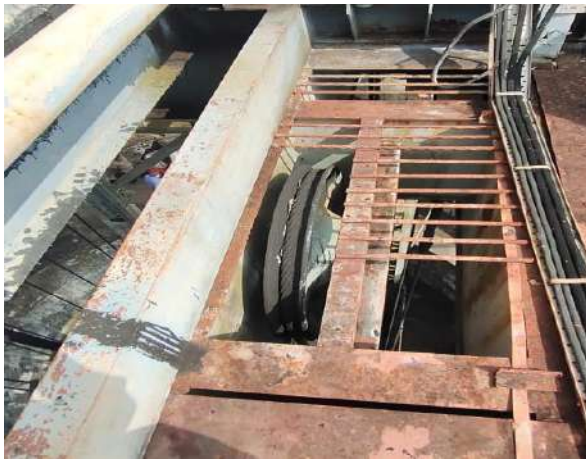
Dried Cardium Compound in Steel Rope of Head Race Tunnel Gate mechanism
