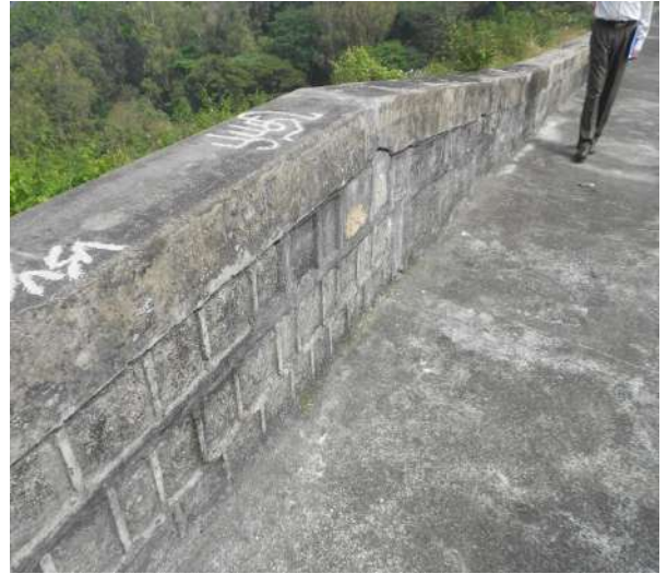
Settlement at the top portion of Dam at Right flank
