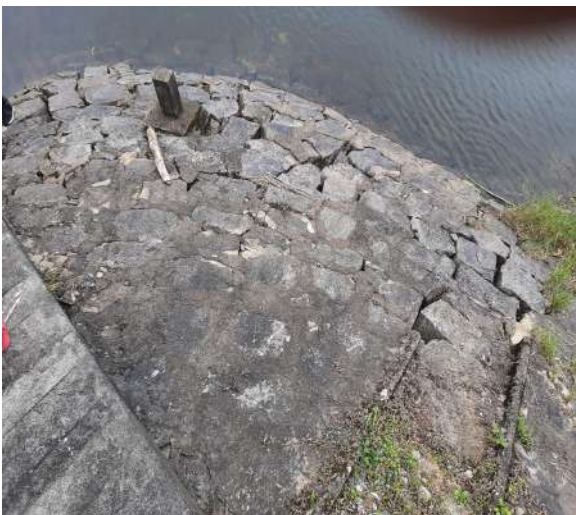
Settlement to CR Masonry Rip Rap at left flank on U/S side of DAM
