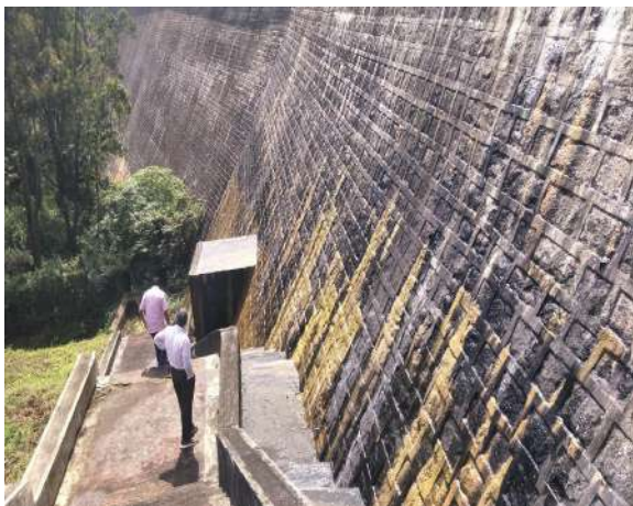
Seepage / Leaching at D/S Left flank
