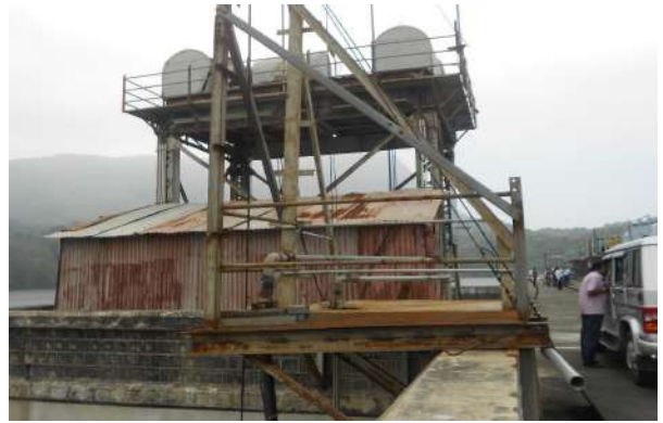
Corroded Scour Vent Structure
