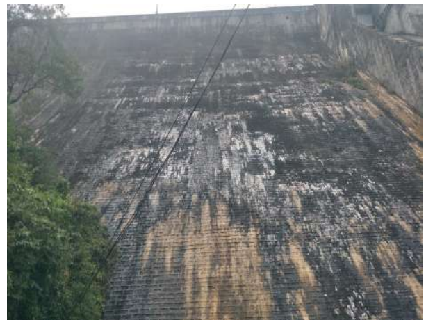
Seepage / Leaching at D/S Right flank
