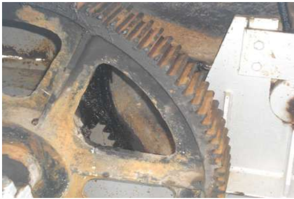
Corroded Scour Vent Hoisting Arrangements
