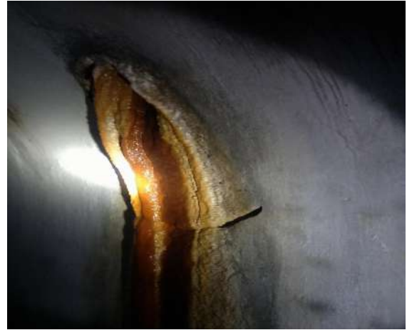
Formation of Calcination inside DG Vertical Shaft
