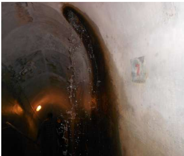
Heavy Seepage in Vertical Shaft No.7
