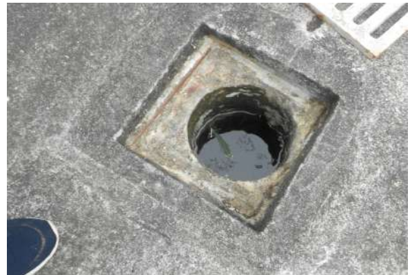
Formation of Calcination inside DG Vertical Shaft
