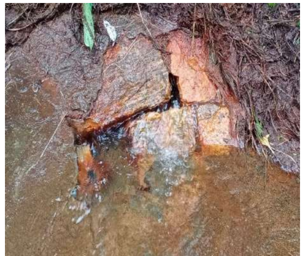
Water Leakage at the right Flank D/S Dam Toe
