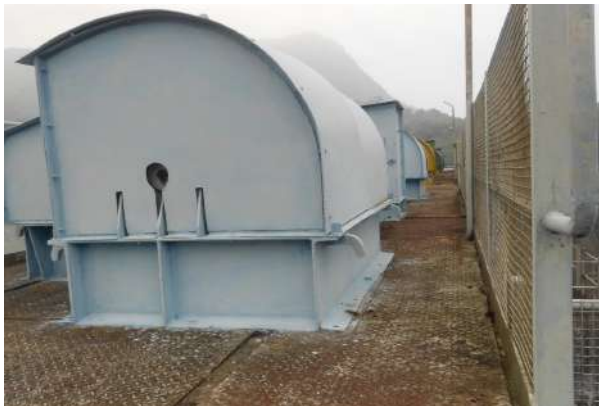
Corroded Chequered plates of Spillway Gates Hoisting Arrangement Platform.
