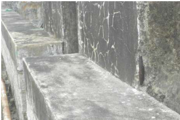
Earth Sludge coming out through Vertical shafts in Blocks 11 & 12
