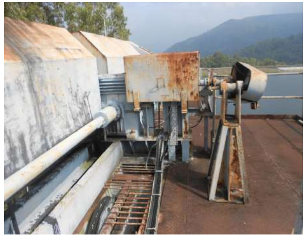
Corroded Chequered Plate and Steel Boxes of Head Race Tunnel Gate mechanism
