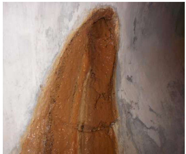
Chocked Vertical Shaft No.14 (View inside Drainage Gallery)
