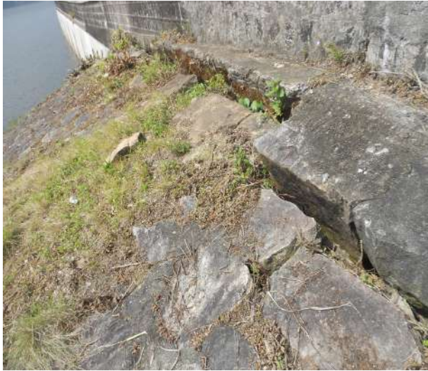
Settlement at Right flank Masonry and Earthen bund junction portion
