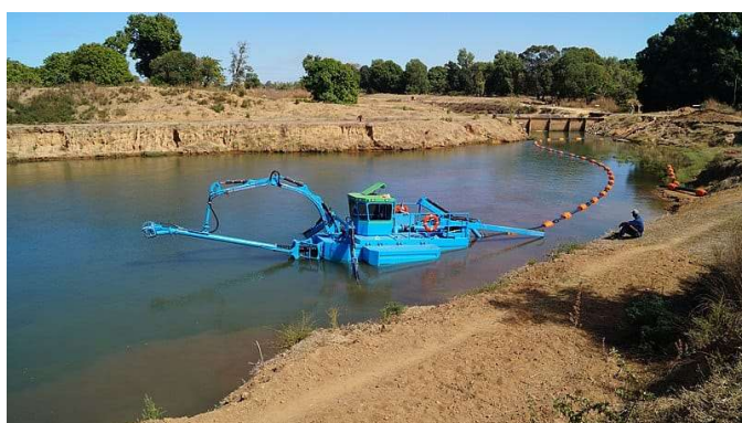
Dredger collecting sediments by using a cutting head, transporting it to geo tubes.
