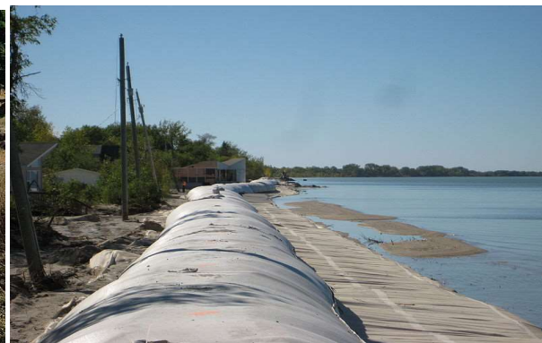
Geotextile tubes being filled with sediments.
