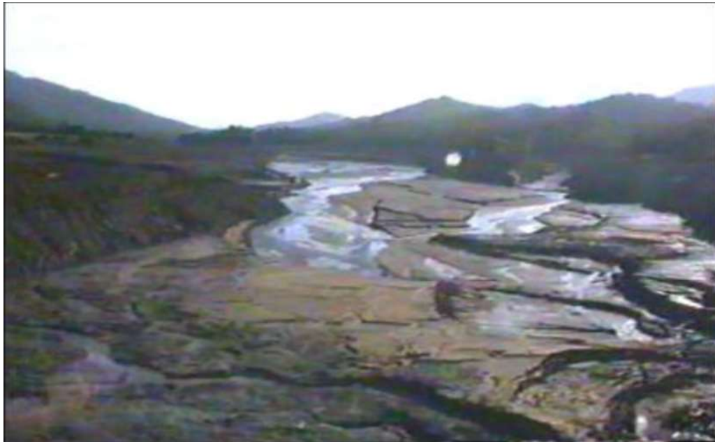
Slit deposition inside Pillur reservoir photographed during 1991
