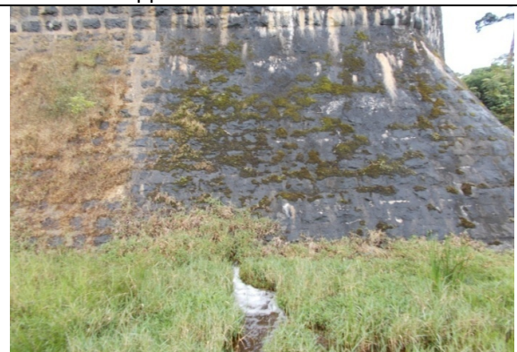
Seepage from drainage saddle dam II (R/F)
