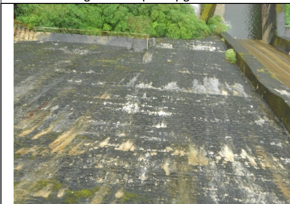
Leakage notice spillway gate bottom
