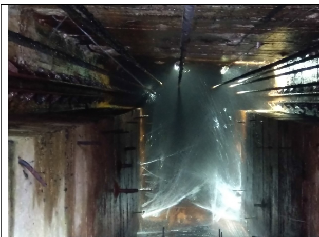
Water jetting inside the Scourvent gate
