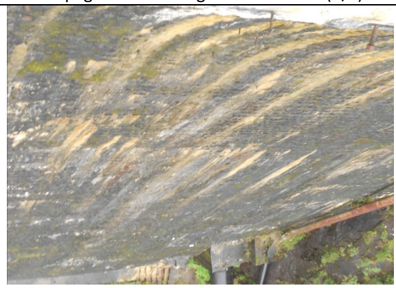
Seepage from drainage saddle dam II (R/F)
