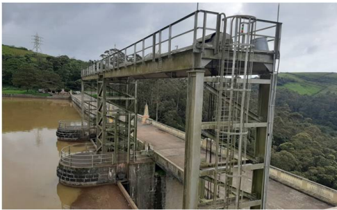
Spillway gate hoisting structure
