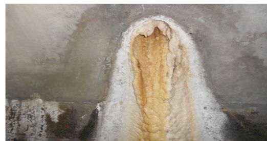
Chocked vertical drainage shafts
