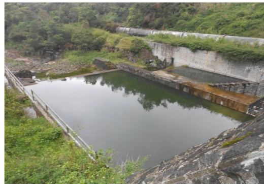
Condition of Spillway and Scour vent stilling basins
