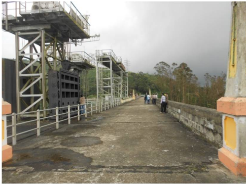
Existing condition of Intake gate hoisting structure
