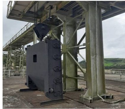
Existing condition of Scour vent Emergency gate
