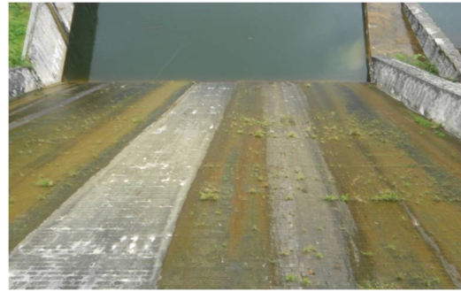
Algae growth and open joints in the spillway glacis
