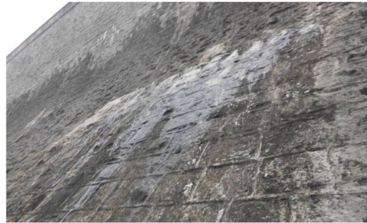
Calcination deposits and sweating on the downstream face of the dam
