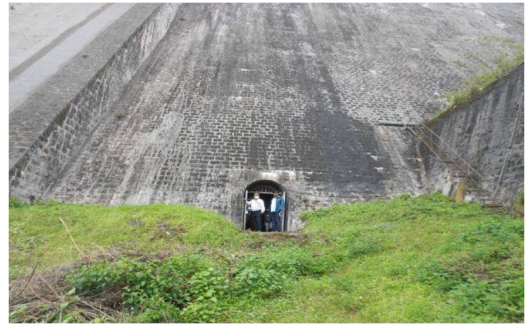
Requirement of masonry steps to assess the drainage gallery
