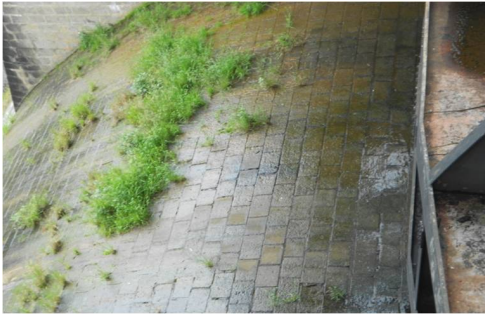
Algae growth and open joints in the spillway glacis
