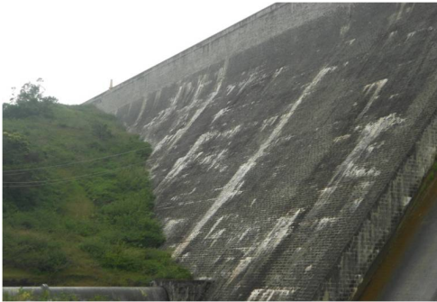
Calcination deposits and sweating on the downstream face of the dam
