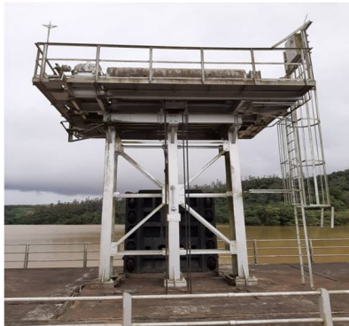
Existing condition of Scour vent Emergency gate hoisting structure
