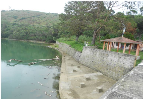
Extension of Slope protection to the left flank side of reservoir
