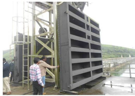
Existing condition of Intake gates
